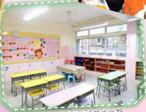
課室已安裝更省電節能的T5光管和貼上濾光熱玻璃膜
